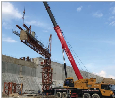
CẦN TRỤC BÁNH LỐP SANY STC800S - 80T WHEEL-MOUNTED CRANE OF SANY STC800S - 80 TONS
